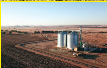
AGI opens three new facilities. p26
