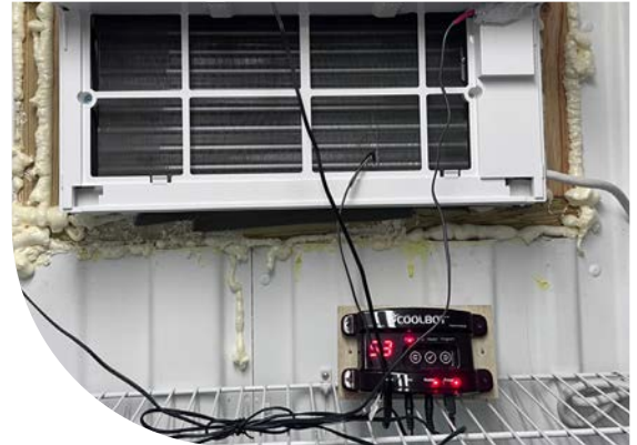
A standard window air conditioner paired with a CoolBot.
