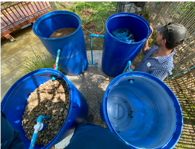
Figure 12. Building a biosand filter. Source: ECHO Asia Staff
