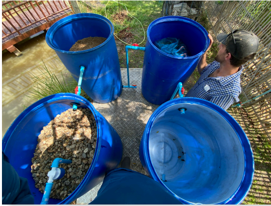
Figure 10. Building biosand filter. Source: ECHO Asia
