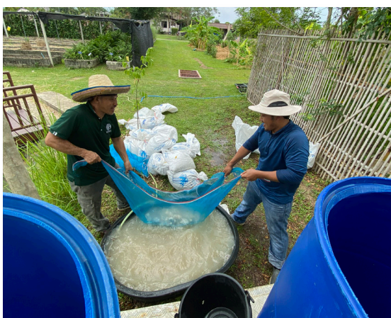
Figure 8. Washing gravel prior to installation. Source: ECHO Asia
