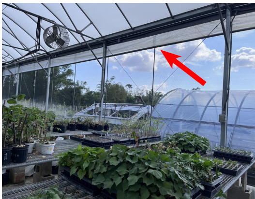
Figure 4. Greenhouse wall with plastic siding that can be partially or completely rolled down to moderate temperature and airflow inside the greenhouse. Source: Tim Motis
